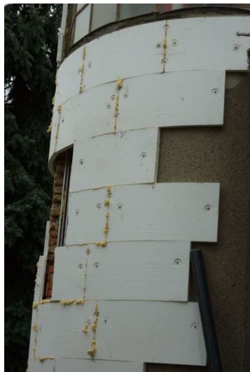
Figures 2, 3: Inappropriate heat insulation of circular sections of building
