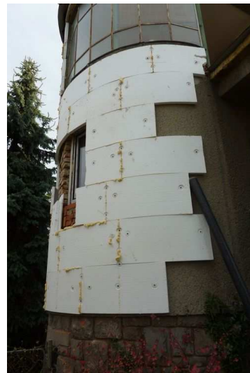
Figures 2, 3: Inappropriate heat insulation of circular sections of building
