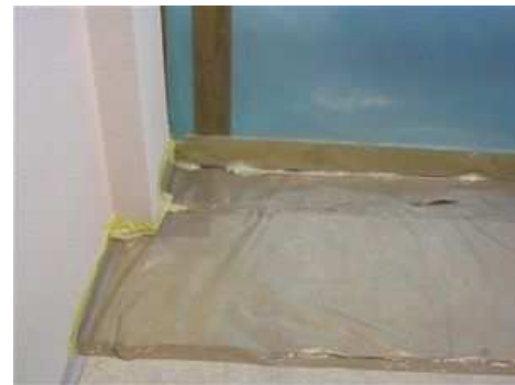
Fig. 1, 2: Controlled area for handling with asbestos products [2]
