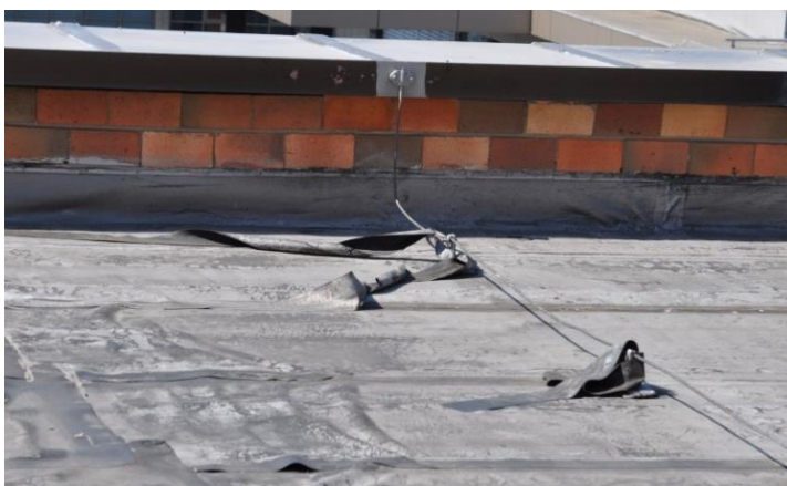
Figure 1, 2: Damaged flat roof waterproofing and rot of the administrative building evaluated in the tab.2
